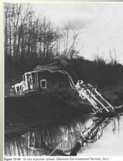
Figure 15-10 In situ injection system. (Harmon Environmental Services, Inc.)
