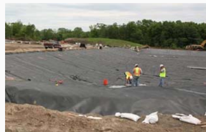
Constructing staging area for sediment.
