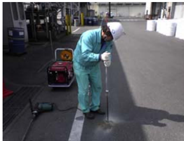
2) Drive a boring-bar into the soil.
