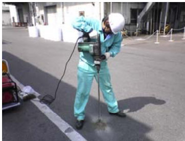
1) Drill a hole through the asphalt with a hammer drill.
