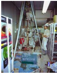
Rotary boring machine
