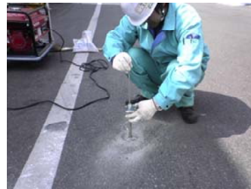
3) Install a guard pipe and a sampling pipe into the sampling bore.
